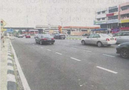
The upgrade of the 1.7km stretch involved resurfacing, upgrading the road kerbs and divider as well as giving it a fresh coat of paint.
